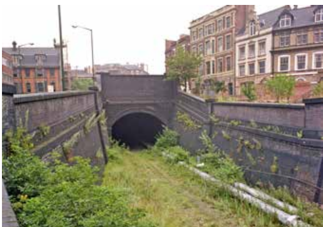
The south portal of Thurland Street tunnel, Victoria Station, 1994. The tunnel currently accommodates steam heating pipes from Nottingham's Cattle Market waste incinerator for the Victoria flats above Victoria Shopping Centre. Photo Nick Catford
